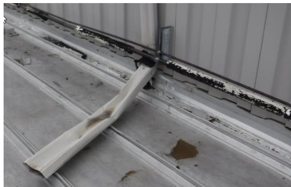
Insulation and drainage damage over Atrium
