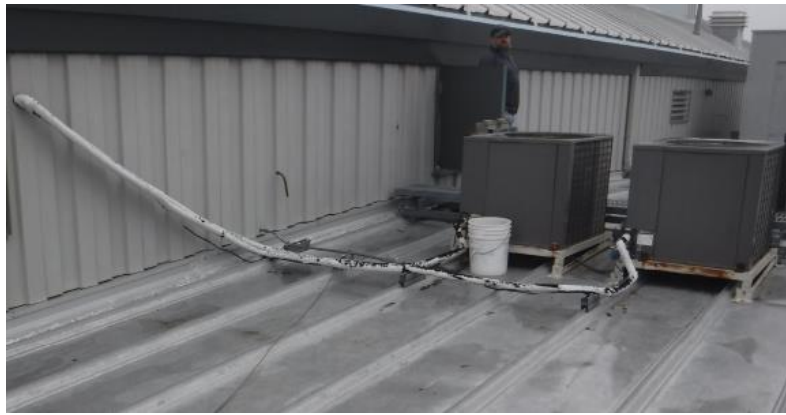
Damage to refrigerant lines over Atrium
