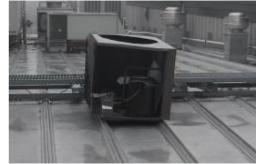
Damaged Condensing Unit over Atrium
